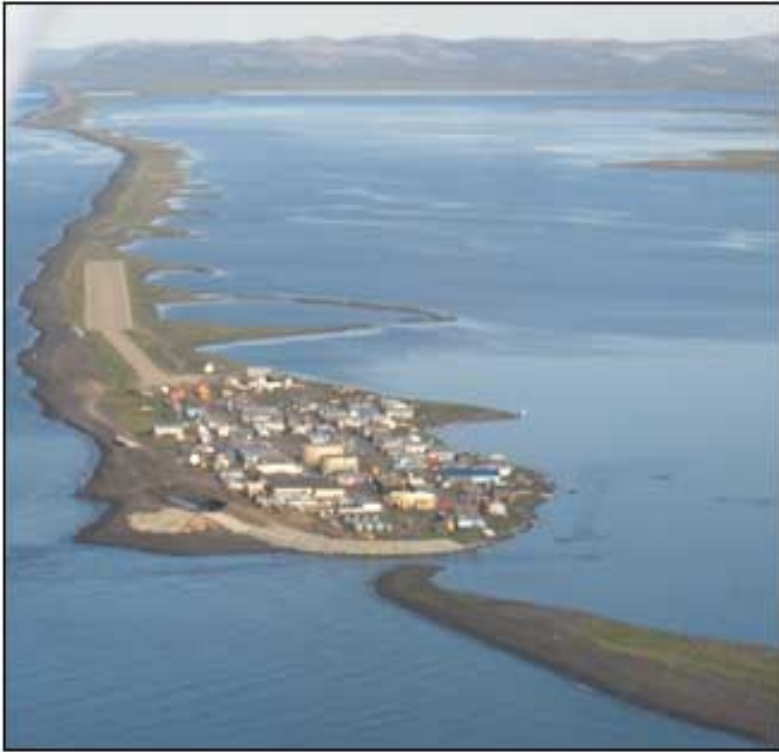
Rock revetment project, Kivalina, Alaska. Source: Millie Hawley, Manager Kivalina Environmental Program
