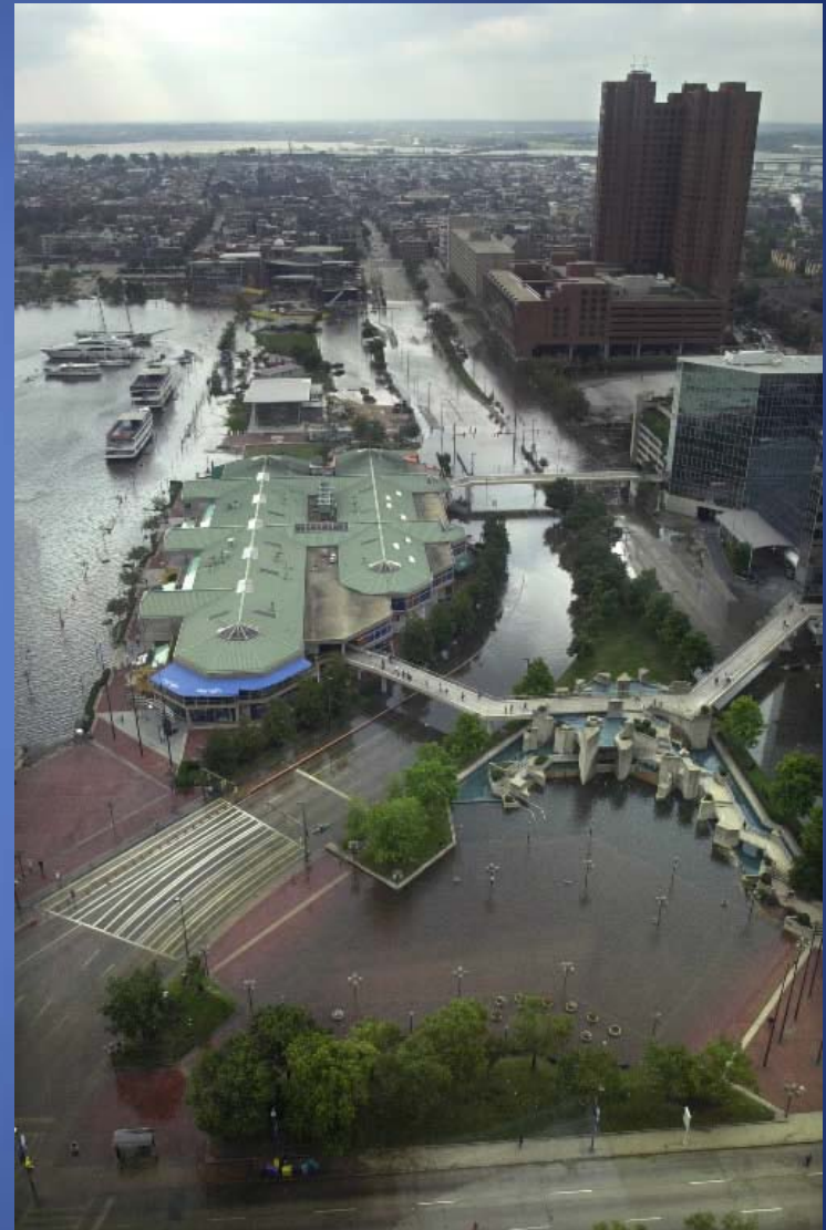
Flooding from Hurricane Isabel 2003
